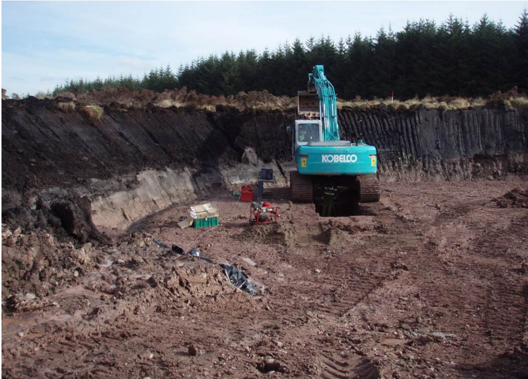
Figure 7-3 Turbine excavation trimmed back to a stable temporary side slope
