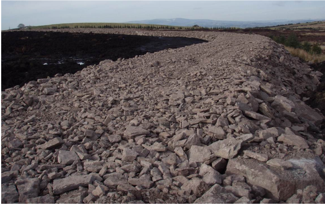
Figure 7-2 Rockfill peat repository on an existing ESB Wind Farm
